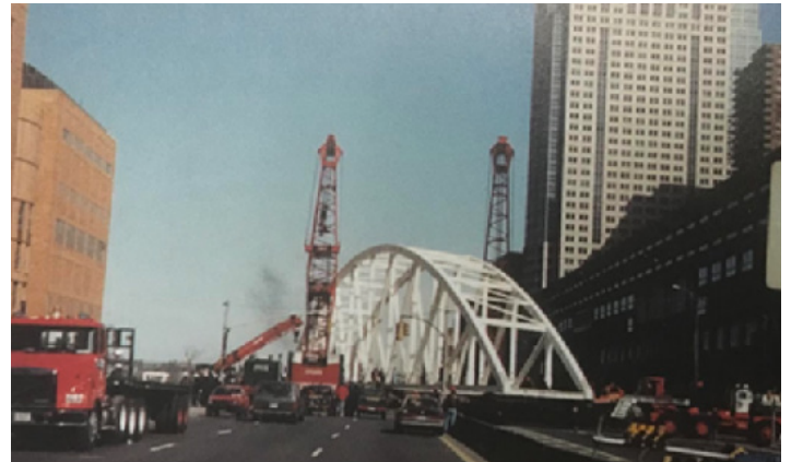
Installing the TriBeCa Bridge
